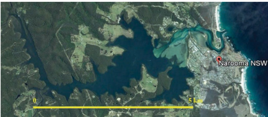
Fig. 10.22 Lake Wagonga, Narooma NSW (Courtesy Google earth). The plan area of the bay is 7 km 2 . The jetties intersect the surf zone, the channel appears deeply scoured and there are significant flood tide sand deltas entering the bay
